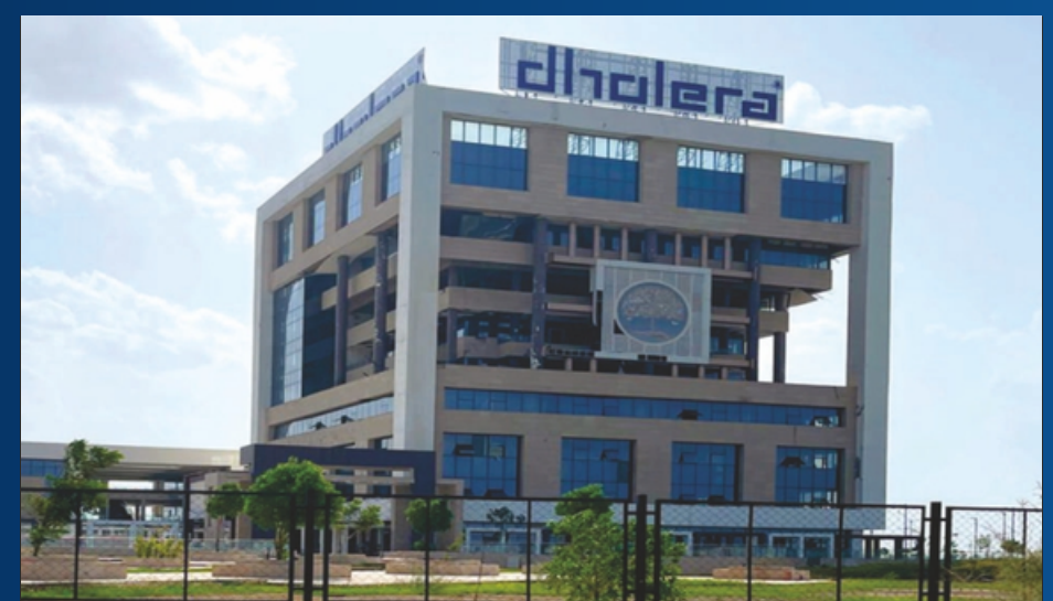
ABCD BUILDING - DHOLERA SIR
